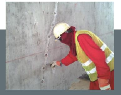
Modern industrial chemistry has developed in a range of single and multi component resisns that can be utilized in the repair of the tunnels, reservoirs, basements, pipelines, lift & escalator pits, structural concrete slabs and elements.
