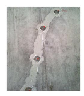
Resin injection is a reparir technique employed to waterproof and repair cracks, voids and defects in concrete and masonry structures.
